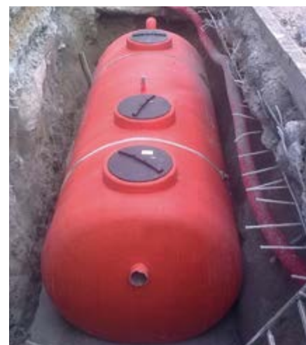
NECOR 30 puerto marítimo
